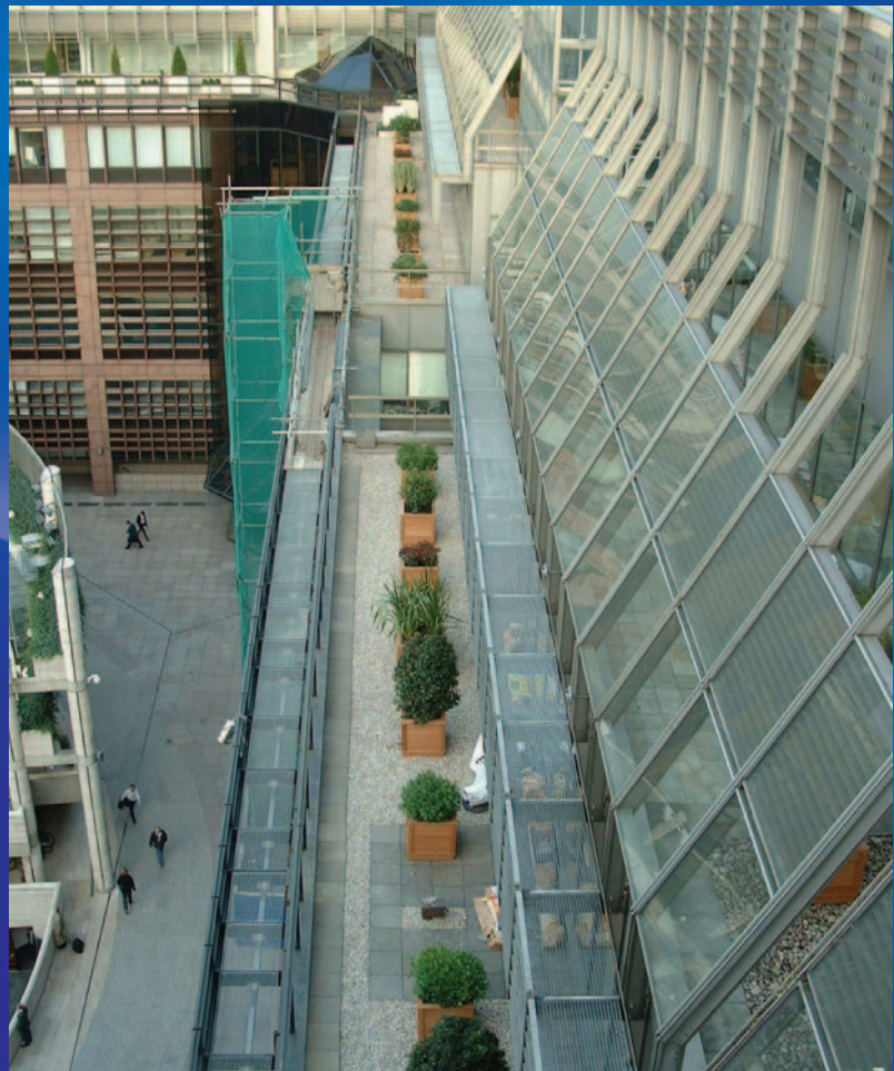
Kemperol 2K-PUR on an inverted roof in central London
