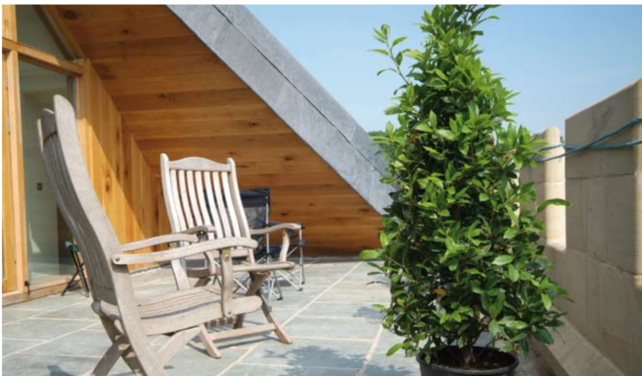
A wide range of hard landscaping materials can be applied directly onto Kemperol for decorative or functional effect, such as this natural slate terrace over Kemperol V210
