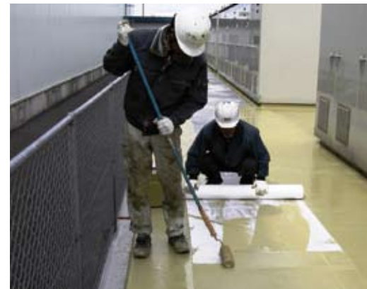
Kemperol waterproofing is applied 'wet on wet', eliminating the need for drying time between coats and allowing large areas to be completed in a single day.
